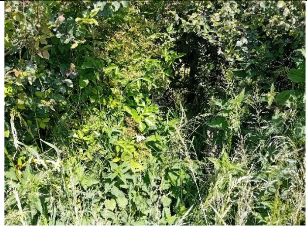
Photograph 14: Mammal underpass on HR3.
