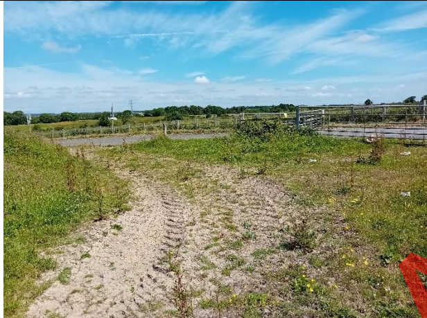
Photograph 9: Example of bare ground on Site. Emergent vegetation is visible
