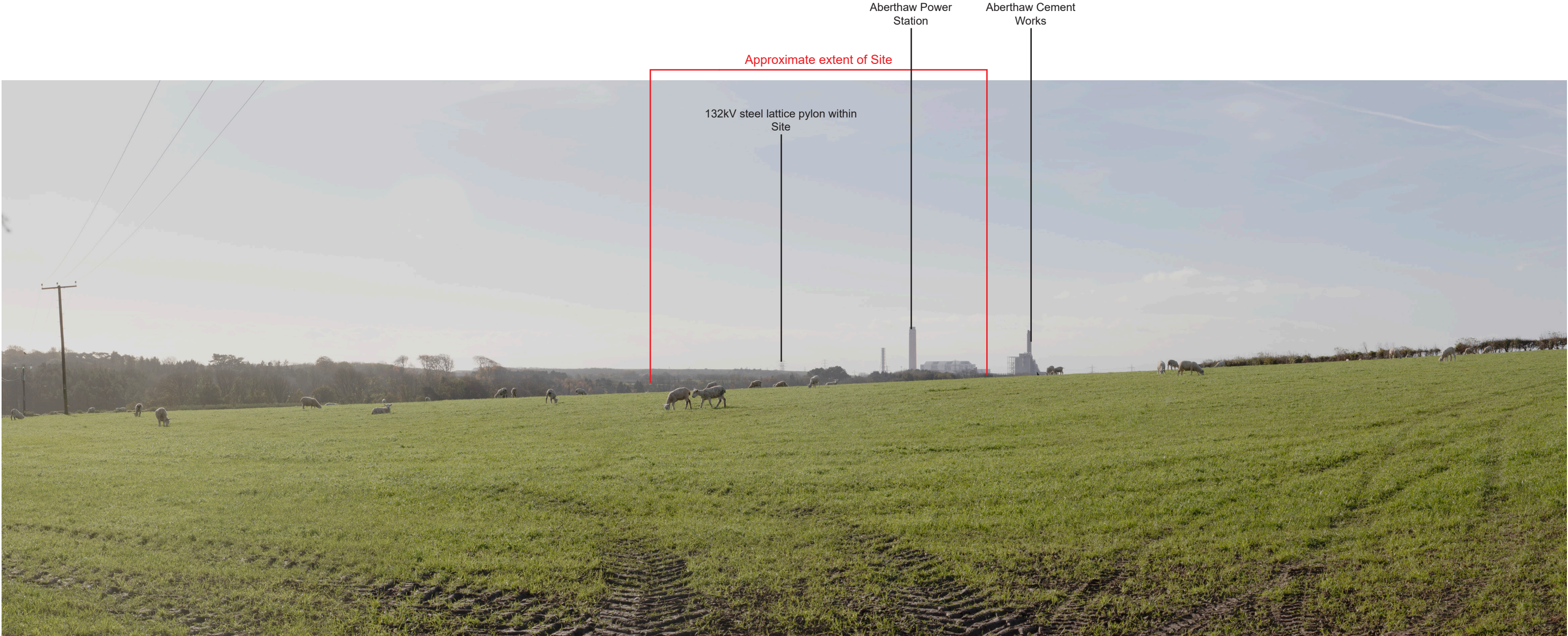
Representative Viewpoint 5 - Unnamed road south of Pancross Farm, to the north east of Site
